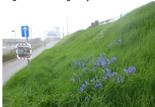
Basin Road North embankment
