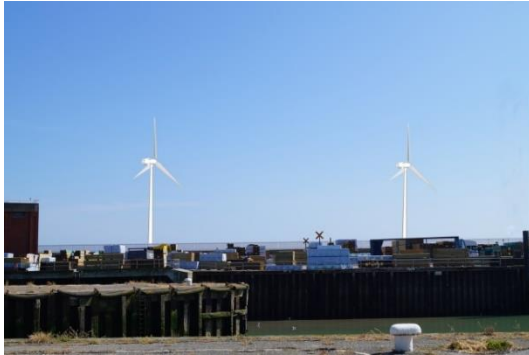
Wind turbines at Outer Layby
