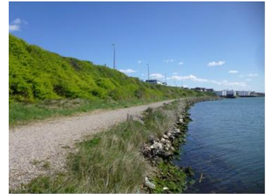
North Canal Bank
